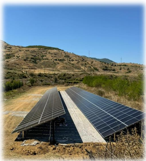
8. Panelet Diellore - Solar Panels
